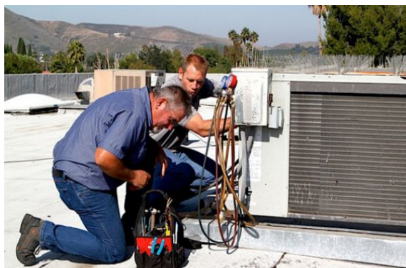
Figure 8: Rooftop HVAC Unit
