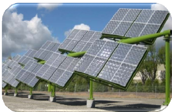
Figure 12: GreenVolts' Concentrating Photovoltaic System Installed in Fremont, California
