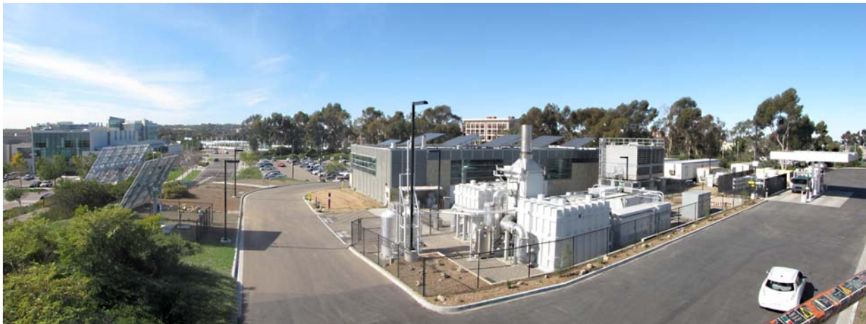
Figure 21: Microgrid Technology Demonstration System Complex, UC San Diego
