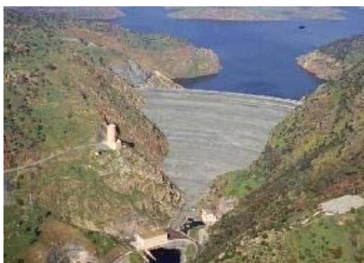
Figure 26: New Melones Dam
