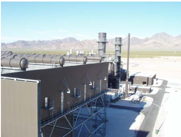
Figure 24: Air-Cooled Condenser
