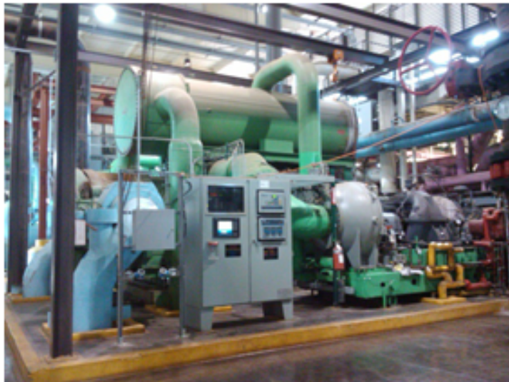
Steam chiller at UCSD campus
