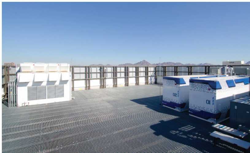
Figure 4. 4,920 servers were deployed in containerized data centers to support eBay's new search engine and its Hadoop clusters. (Source: eBay photo, used by permission)
