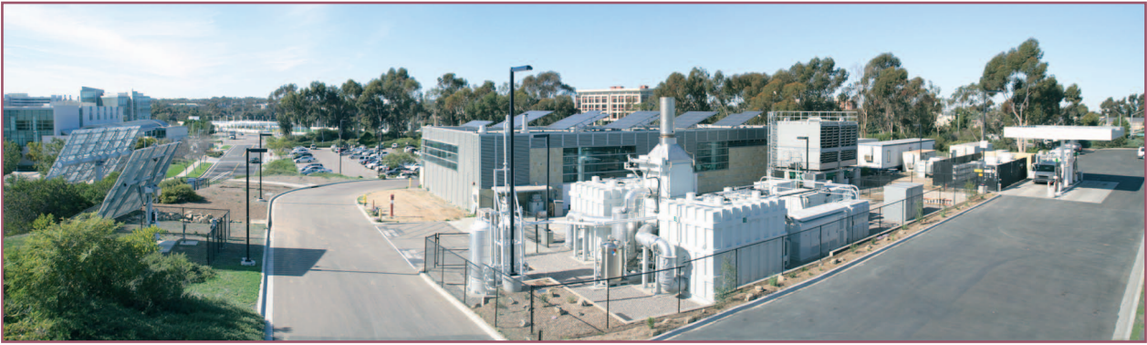
figure 3. UCSD's 2.8-MW fuel cell, which utilizes biogas fuel (used with permission).
